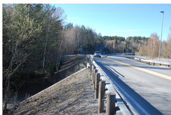
Figur 3-24 Kulvert under fv. 353
